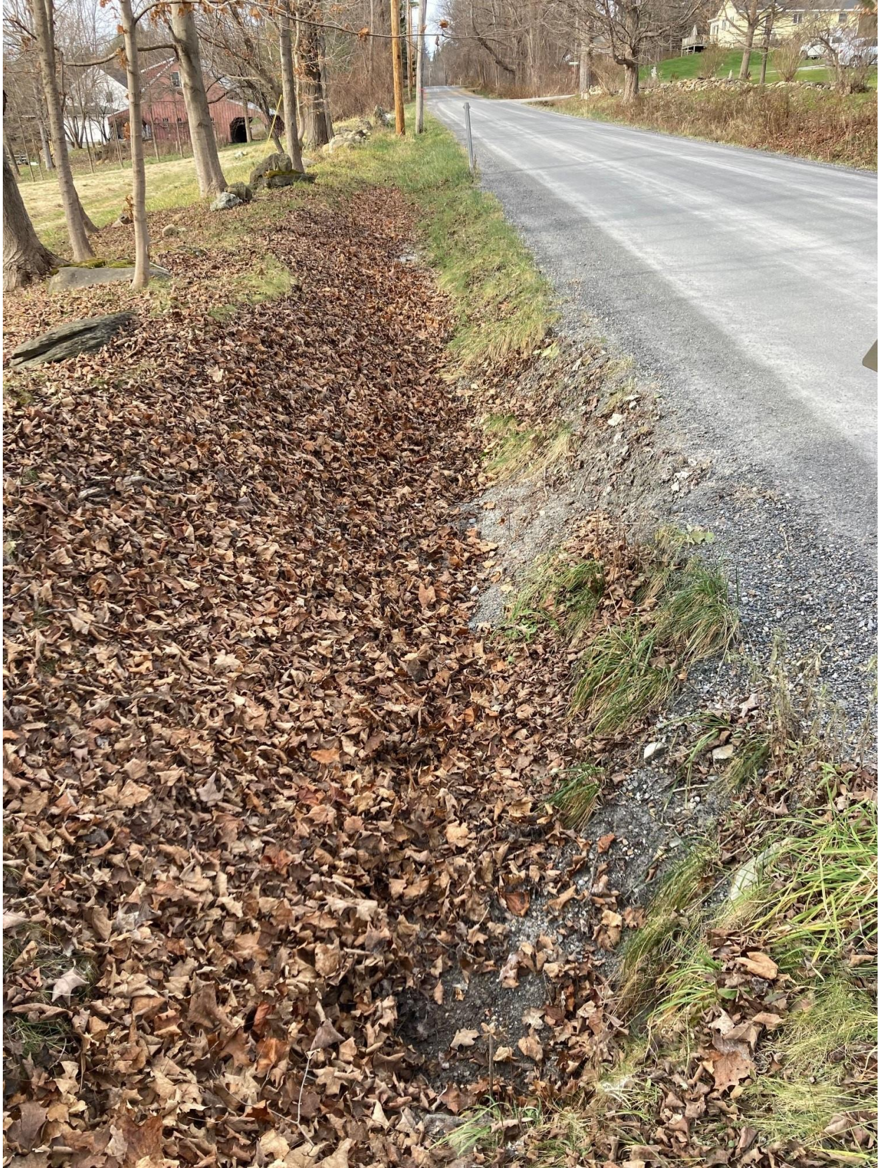
Figure 5 Segment 30793 Ditch 2 Before
