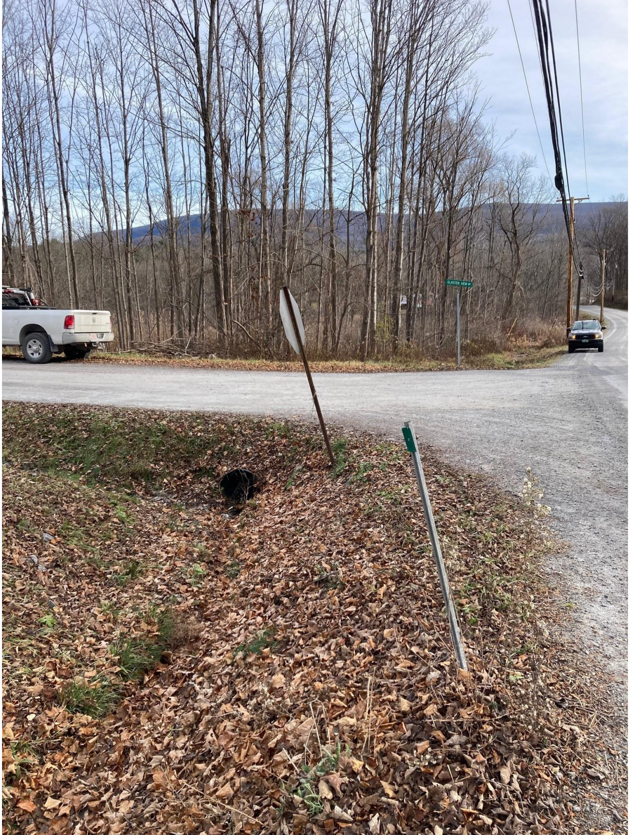
Figure 1 Segment 102860 Culvert Before
