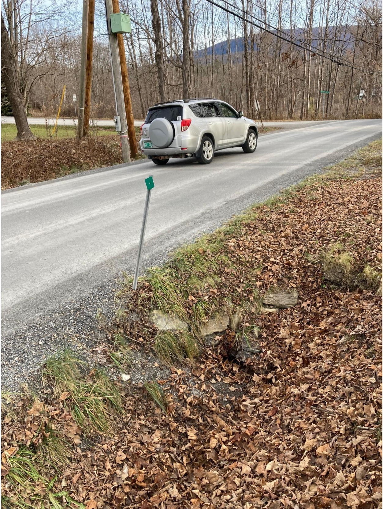
Figure 3 Segment 30793 Culvert Before
