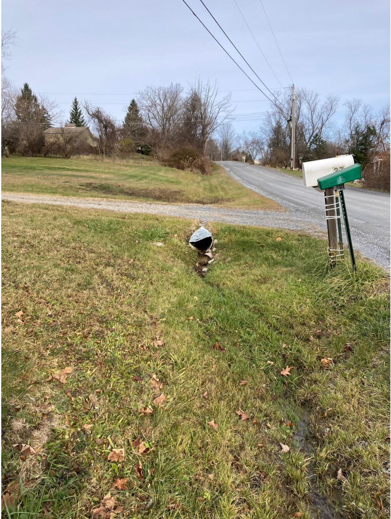
Figure 2 102860 Driveway Culvert and Ditch Before
